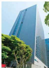
MS&AD Holdings Head Office Building
